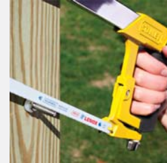
Step 2 Cut thread flush with nut.
